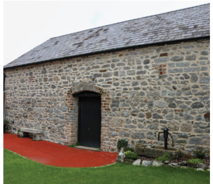
Caretaker's shed restored.
