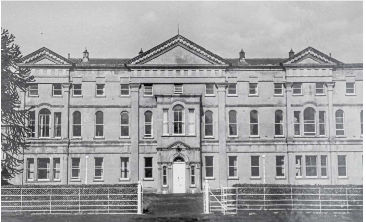
1903: The Front House, hiding the old, provided the familiar façade for Knockbeg for the next 120 years.
