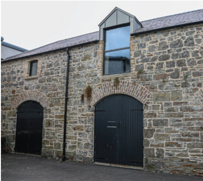
Original coach house restored.
